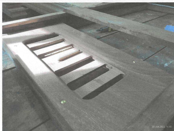
New Hit 'n' Miss ventilator grill Copied from the original.
