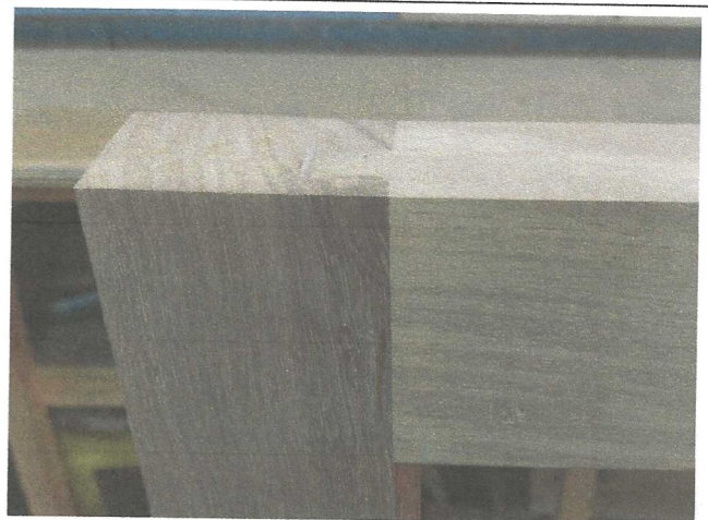
Window cleaned with 180 grit sandpaper. Prepared for painting.
