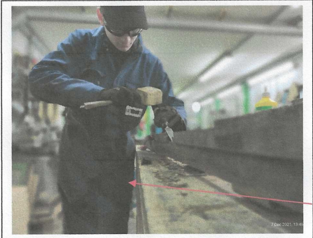
Removing Decay from the latch placement
