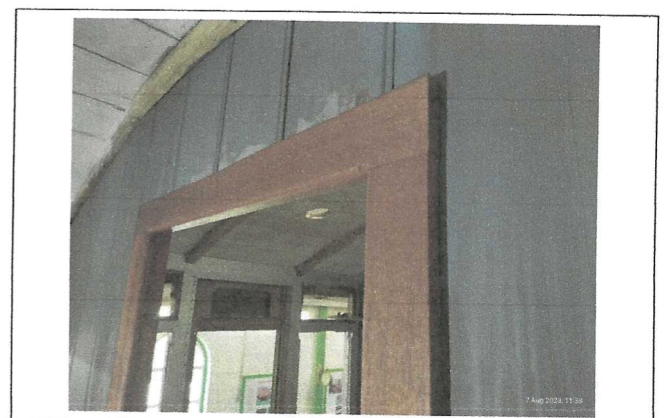
Fitting frame to compartment wall
