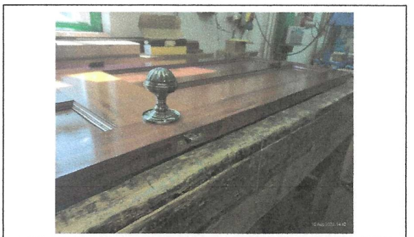
Latch & doorknob fitted
